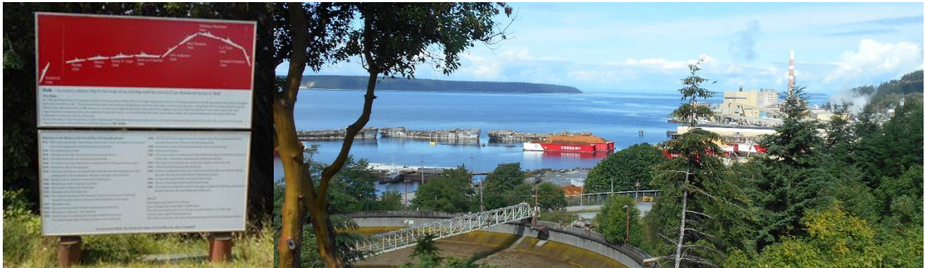
How they made a floating break water using old merchant and war ships
