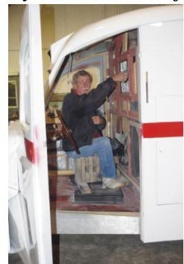
Keith cleaning up window frame.
